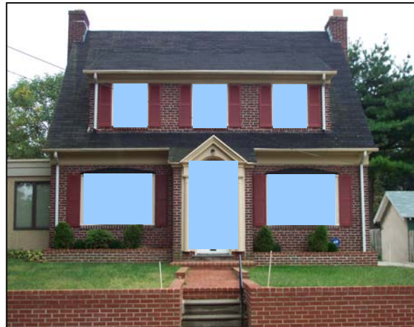
This traditional building has a wall to opening ratio of approximately 1 to 1.
